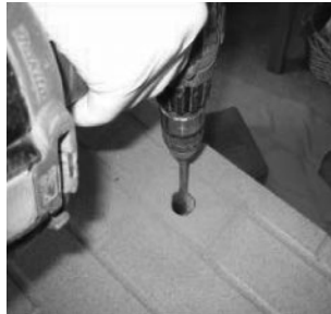
Drilling a Hole for the Gas Line
