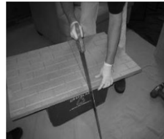
Cutting the Panel to Size
