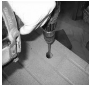
Drilling a Hole for the Gas Line
