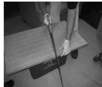
Cutting the Panel to Size
