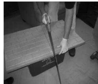
Cutting the Panel to Size
