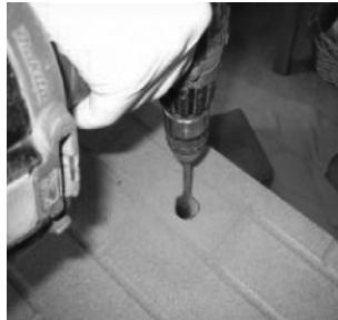
Drilling a Hole for the Gas Line
